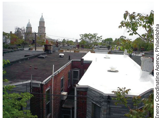
Figure 11: Cool Roofing on Urban Row Homes
