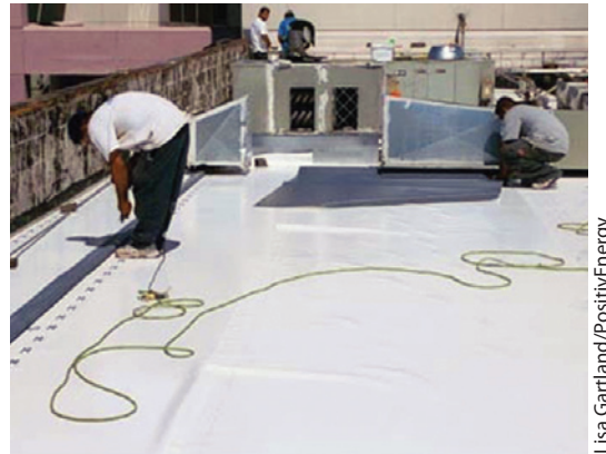
Figure 14: Installation of a Cool Single-Ply Membrane
