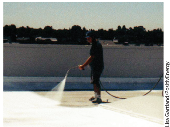
Figure 7: Cool Coating Being Sprayed onto a Rooftop
