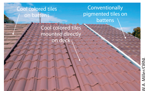
Figure 8: Conventional and Cool Colored Tiles
